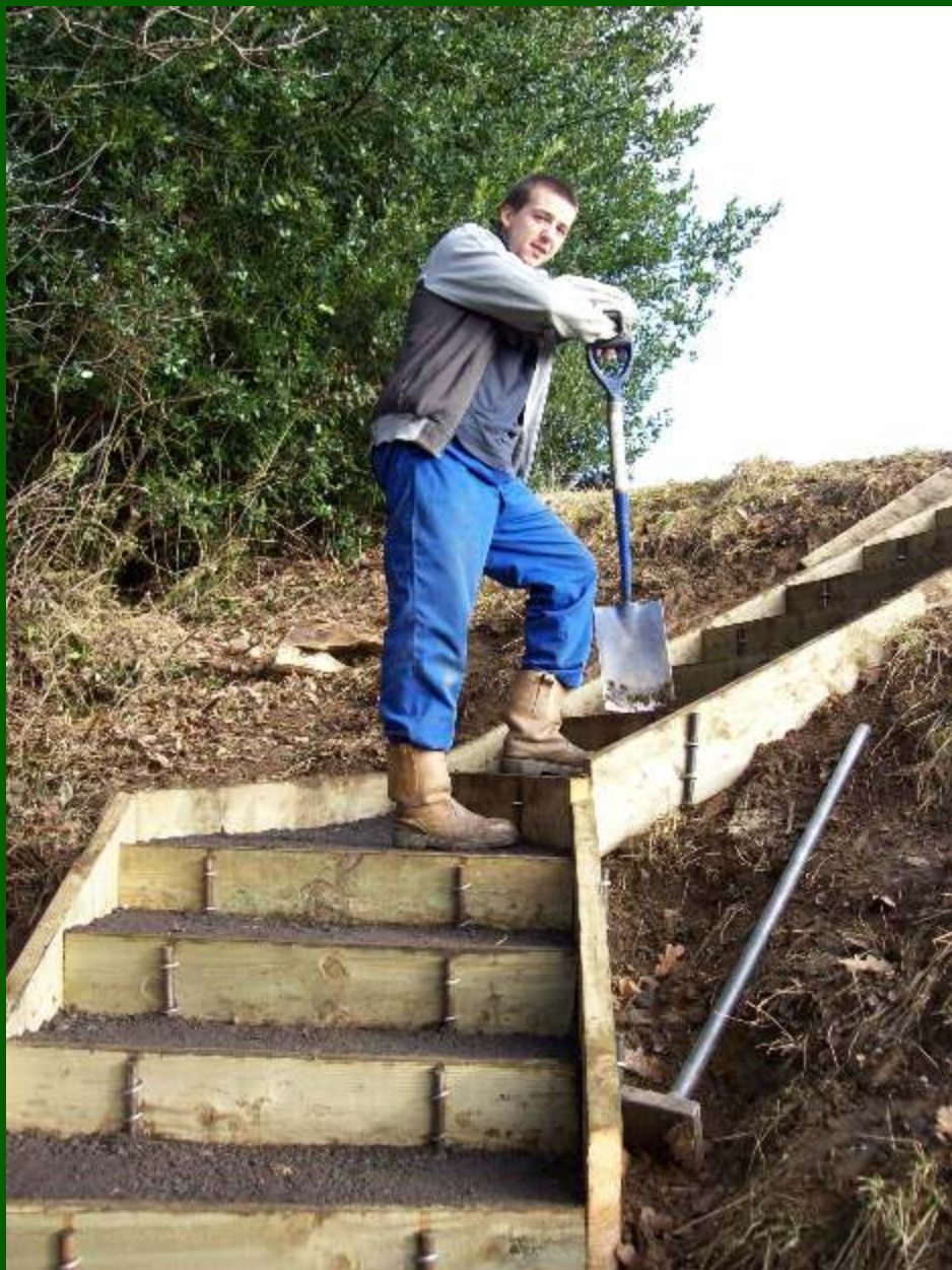
Construction of Steps at Holdworth Farm (??FP No??)
