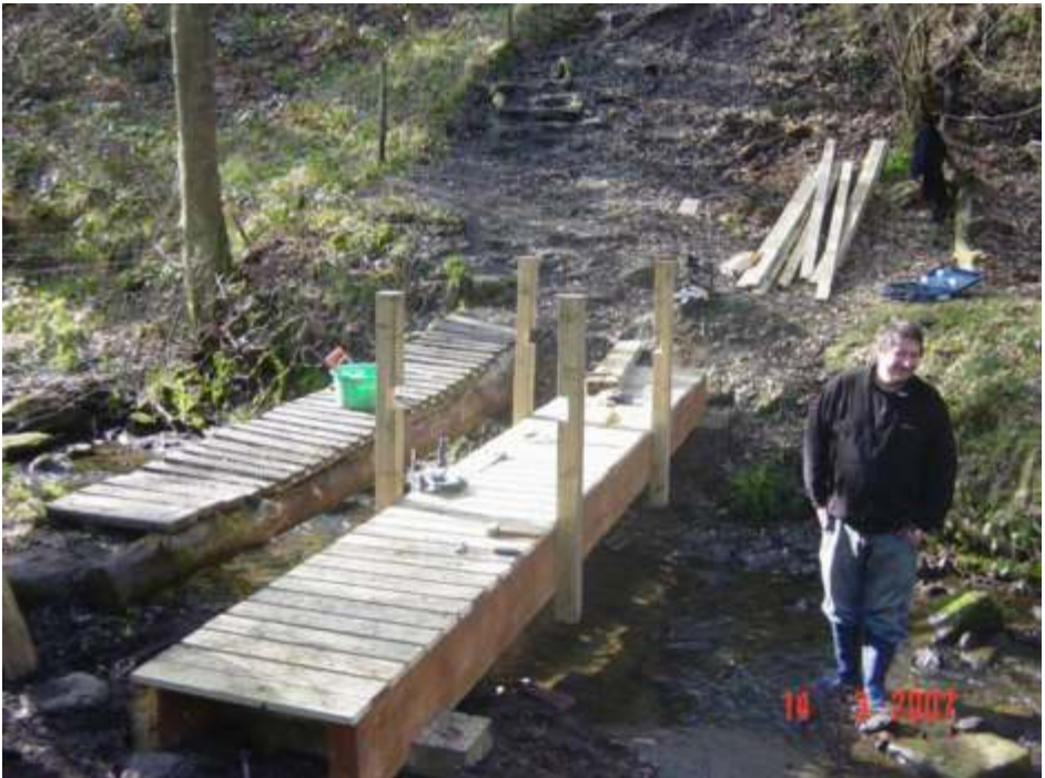
Replacement Bridge on Holmfirth FP168
